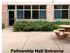
Fellowship Hall Entrance
